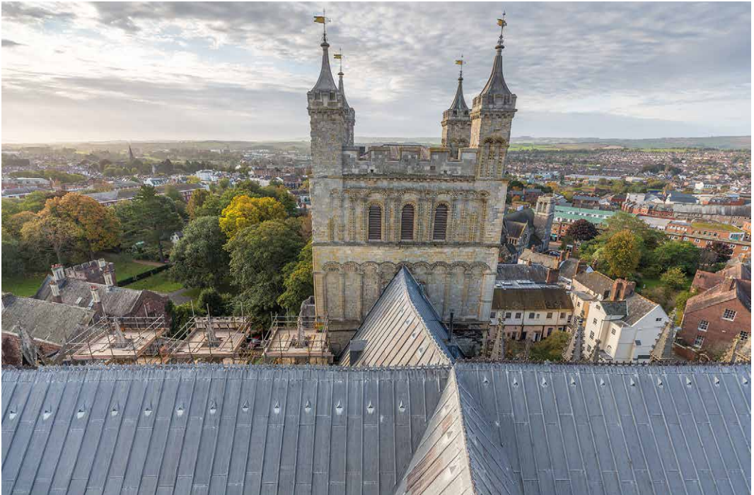
↑ Figure 4. Lead roof of Exeter Cathedral, view from the North Tower to the South Tower (Photo © T. Pestridge, Exeter Cathedral; image modified).
