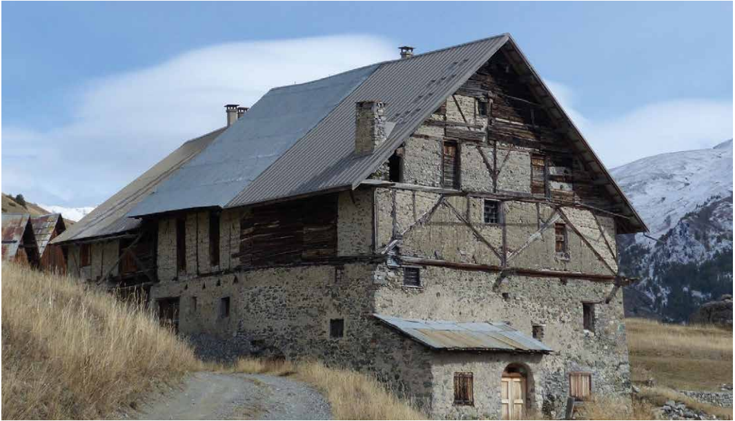
↑ Figure 2. An alpine house (at 1900 m altitude) for a single family, dating back to at least the 18 th century. Different types of timber construction were used for the upper floors: half-timbering and Blockbau (Photo by L. Shindo; image modified).
