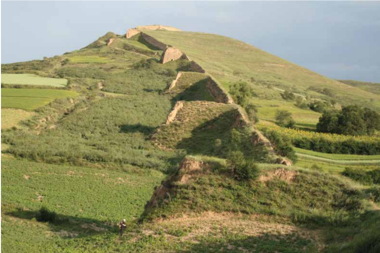
Figure 2. The horse faces on the Wall, Shuozhou, Shanxi (Great Wall Resource Survey Shanxi Team I).
