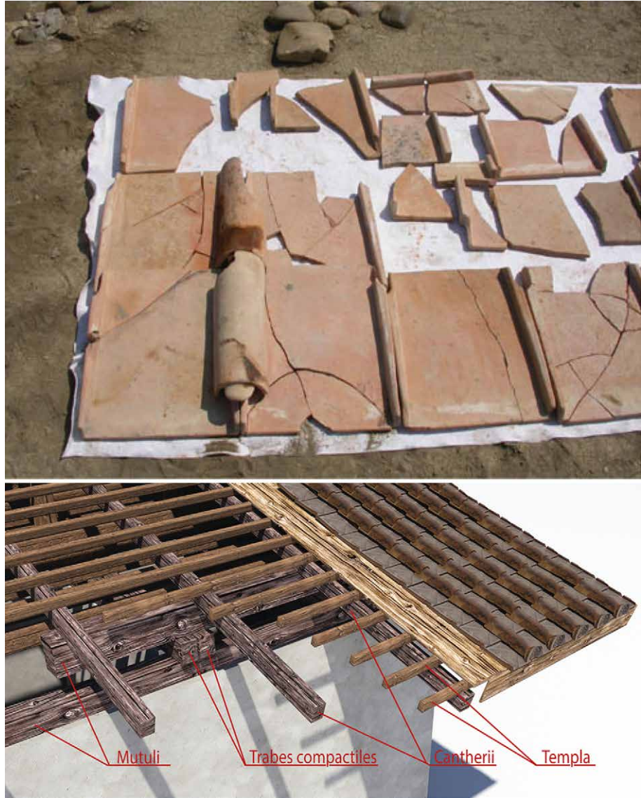
Figure 8.8. Tiles found in the Temple of Tinia and virtual reconstruction of a roof (after Garagnani et al. 2016b).
