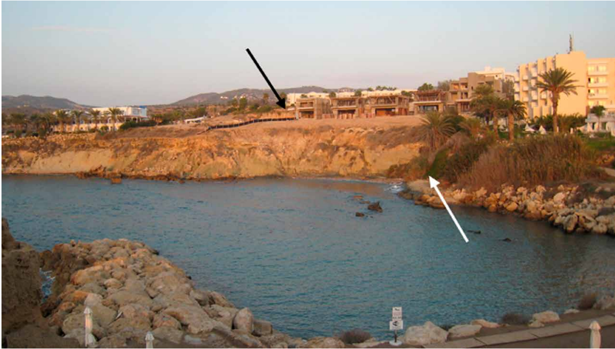
Figure 6. The coastal cliffs at Kissonerga Mylouthkia. View to the northeast. Location of the Neolithic wells (black arrow) in relation to natural water springs in the bay below (white arrow). Note the rapid build-up of urban development at the site compared to the photograph taken in 2004 by Galili et al. (p. 98, fig. 8.3) (Photograph by Duncan Howitt-Marshall, 26 October 2017).
