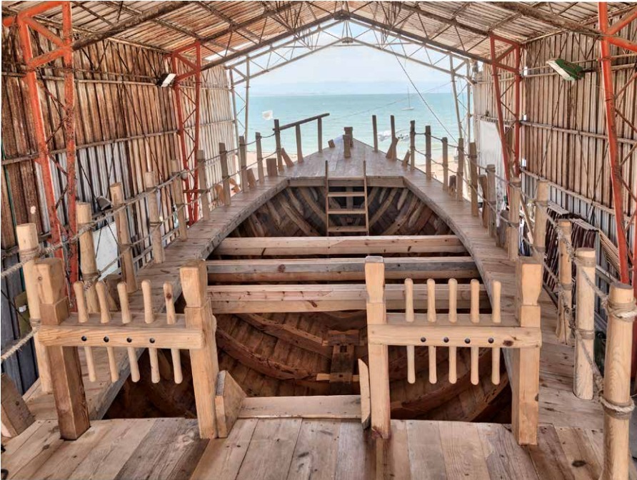
Figure 9. A view from stern to bow during construction showing the slightly cambered decks and the walkways connecting them. In the rectangular opening in the hold the crossbeams and mast step can be seen. The extended futtocks and top-timbers serve for the rails and as a base for bits for hawsers or mooring lines (Photo A. Efremov).
