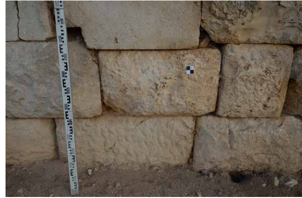
Figure 18. The Late Antique City Wall, re-used ashlar blocks from the Hellenistic city wall (@ Patara Excavation Archive).
