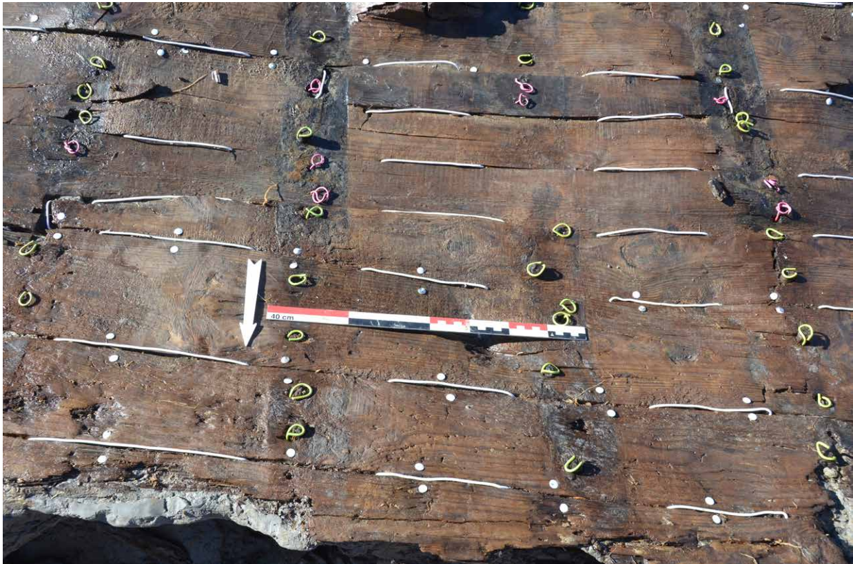
Figure 15. Repaired strakes fastened to the frames with nails highlighted in pink (Copyright Julie Labussière).
