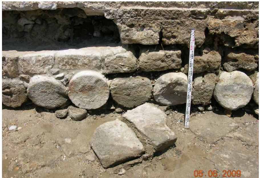
Figure 6. East-West view of the Ottoman seawall foundation made of a row of columns in secondary use placed on top of the Hellenistic docking platform floor (Photo: J. Sharvit).
