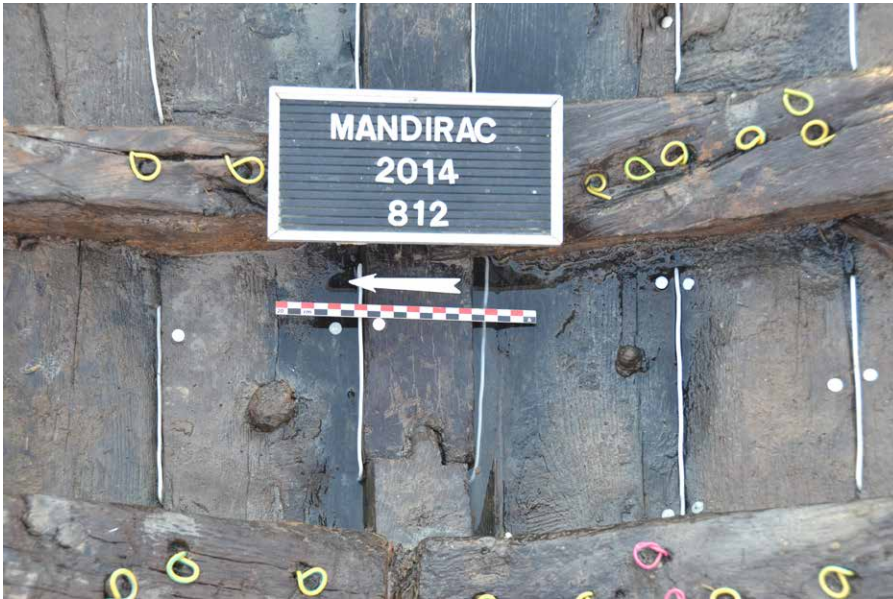
Figure 6. Treenails in the garboard planks used to plug holes (Copyright Julie Labussière).
