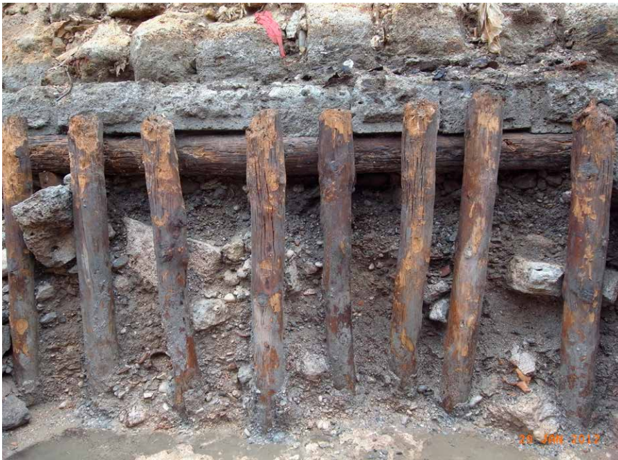
Figure 12. A row of wooden posts and beams that served as a foundation for the Ottoman seawall. The first row of stones was laid directly on top of the wooden beam. In some cases, the posts penetrate through all the layers into the bedrock (Photo: J. Sharvit).
