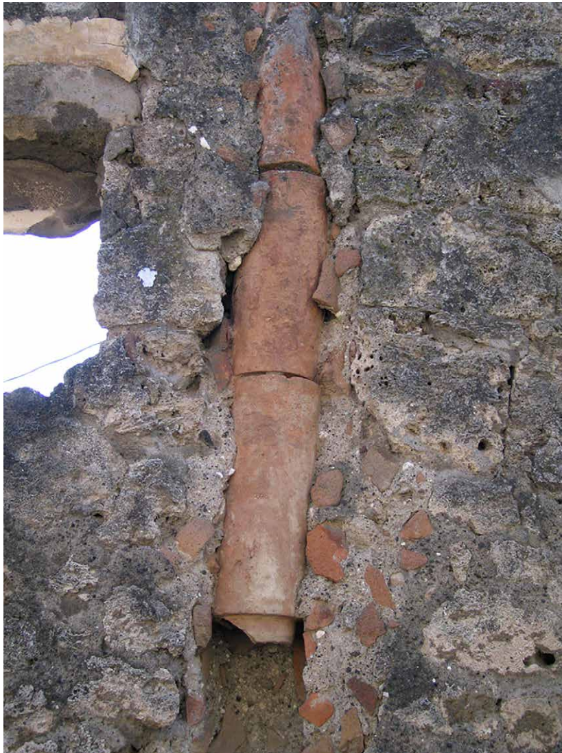
Figure 4. Pompeii, terracotta downpipe (Photo: Koloski-Ostrow).
