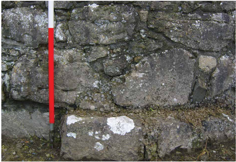
Figure 1. Clones, County Monaghan, is a Type 1 round tower with poor masonry quality (Source: Kerr 2011).
