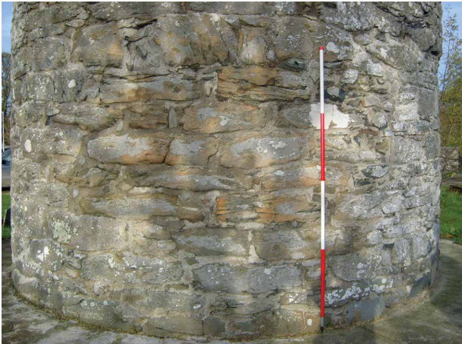
Figure 2. Inishkeen, County Monaghan, is a Type 2 round tower demonstrating an improvement towards ashlar as the medieval period develops (Source: Kerr 2011).
