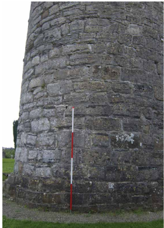
Figure 4. Glendalough, County Wicklow is an example of a Type 4 round tower with near-ashlar masonry (Source: Kerr 2011).
