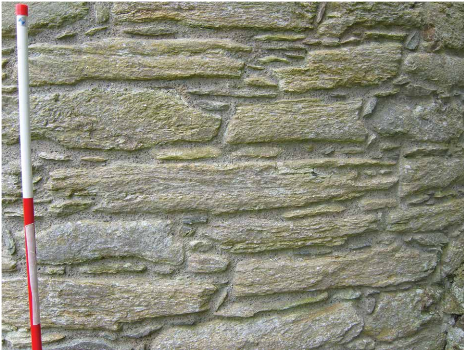
Figure 3. Type 3 round tower Armoy, County Antrim, demonstrates the development towards ashlar masonry with an improved masonry quality from Type 2 (Source: Kerr 2011).
