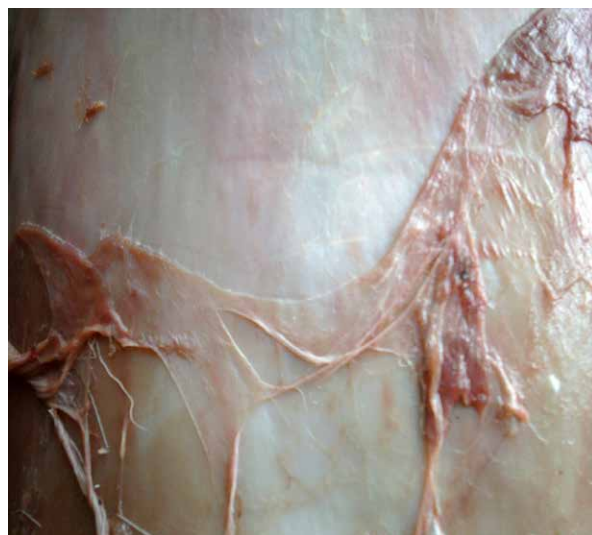
Figure 4.3-2. Membrane Removal wet scrape method.
