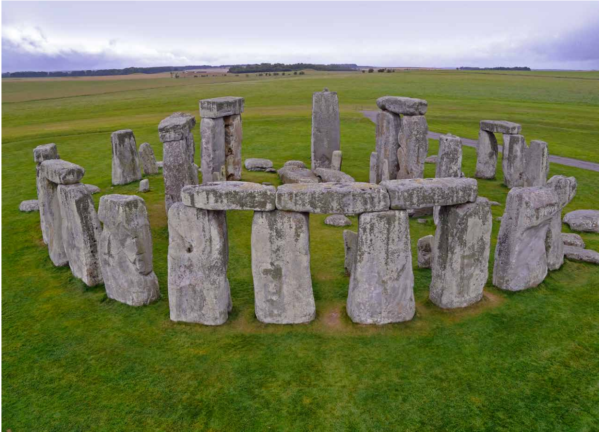
Figure 6.4. Stonehenge viewed from the northeast
