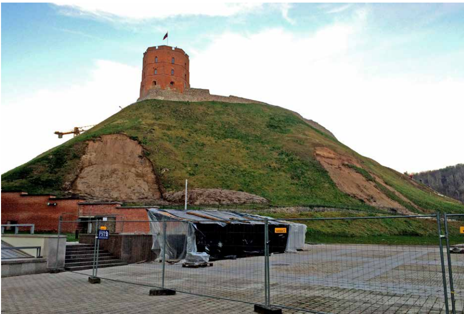
Figure 7. The landslides on the south-west and south slopes of Gediminas Hill in 2017 (E. Povilaitytė-Leliugienė).
