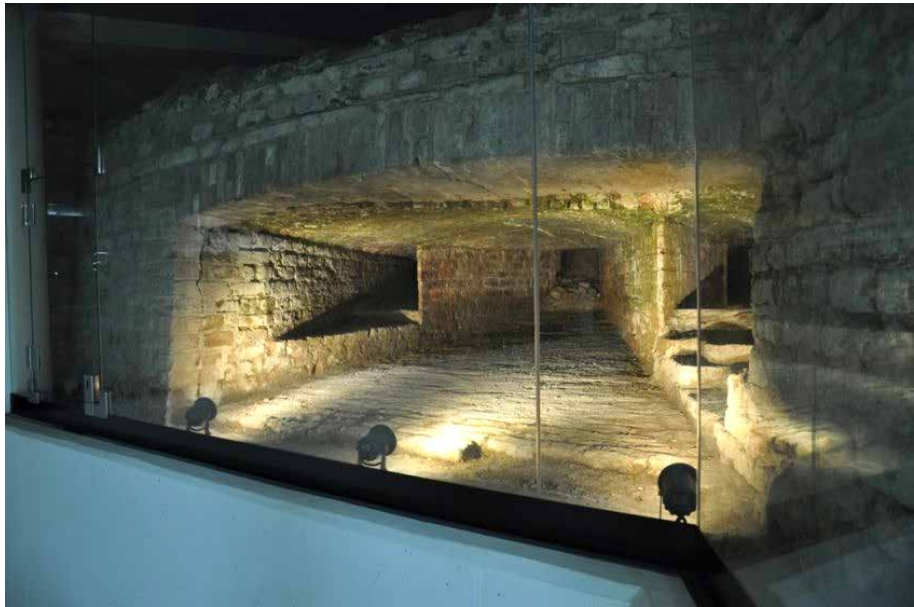
Figure 4. Fire tube in the north-eastern tower ( www.cu2030.nl ).
