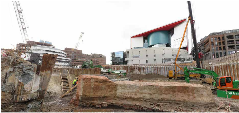
Figure 5. Figure 5. The Main gate before dismantling (Source: www.cu2030.nl/G . Serné).
