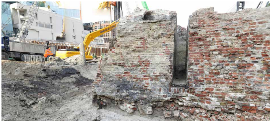
Figure 8. The south-west tower before dismantling ( www.cu2030.nl/ ).
