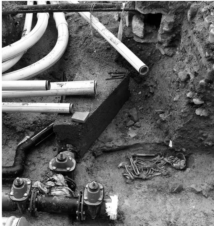
Figure 9. Grandson view of trench excavation (Archeotech SA).
