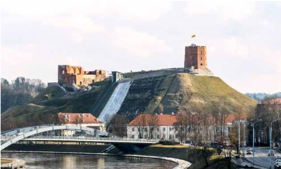
Figure 6. The landslide on the north slope of Gediminas Hill in 2017 (E. Povilaitytė-Leliugienė).
