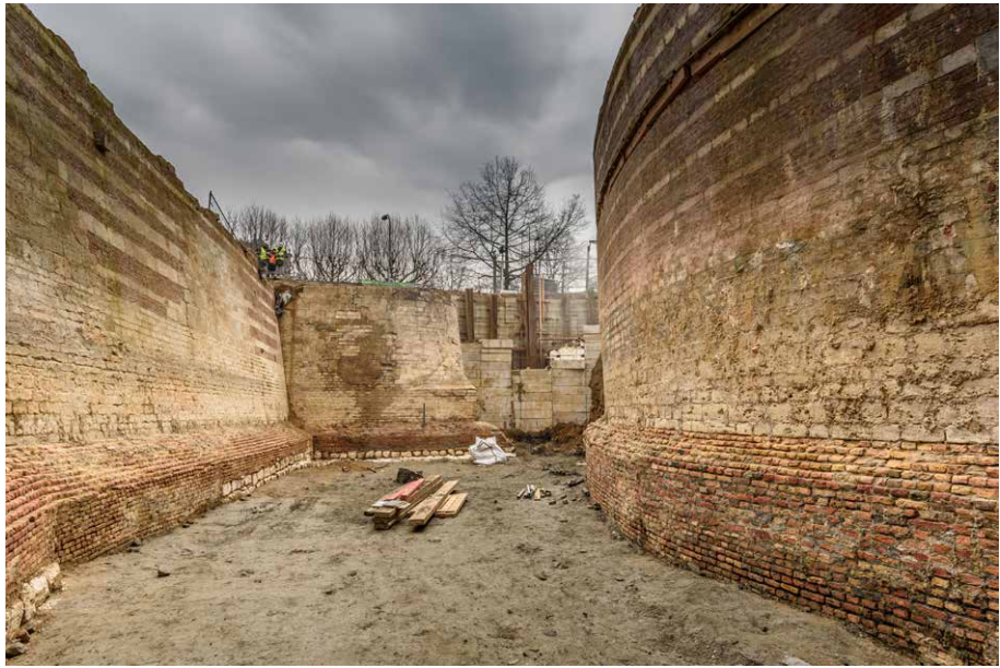
Figure 3. View from the west of the excavation of Kipdorp site with the monumental city walls of the bastion, the orillon and bridge (Koen Ver Eecke).
