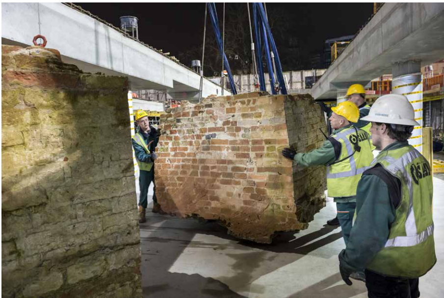
Figure 6. The main gate blocks during replacement ( www.cu2030.nl/G . Serné).
