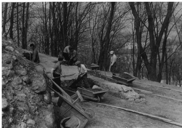
Figure 2. Workers removing earth from the ancient masonry structures in 1940 (E. Povilaitytė-Leliugienė).
